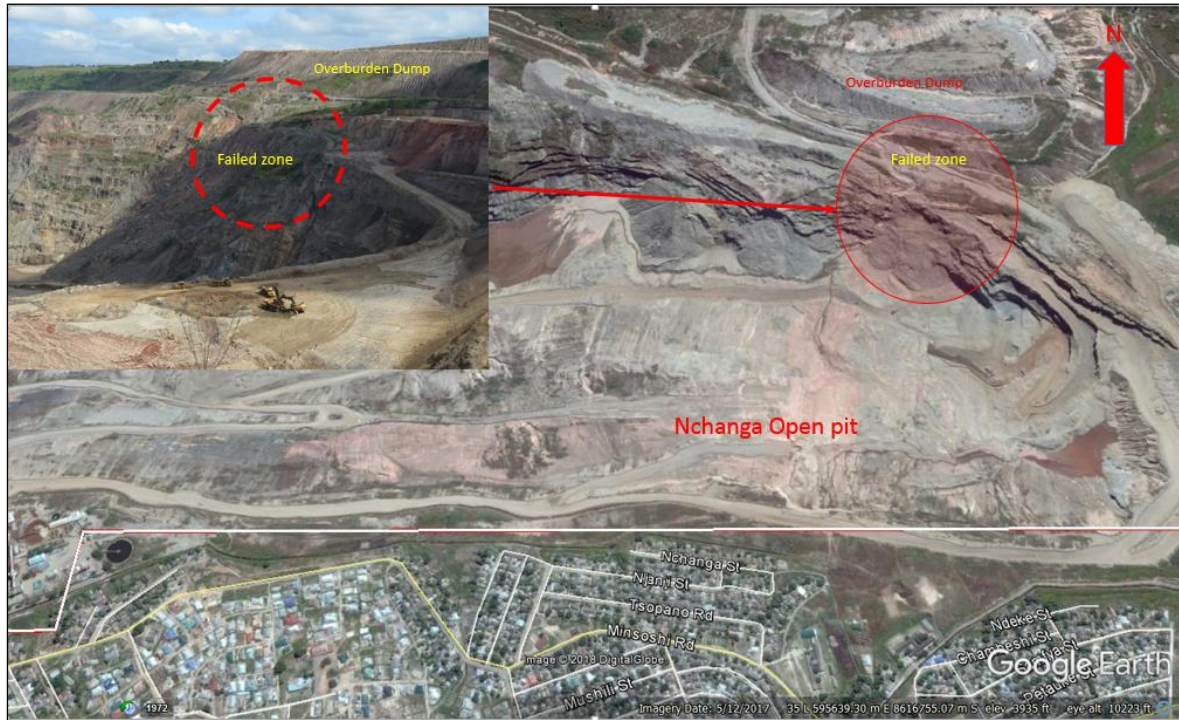
Figure 1: Nchanga Open Pit failure zone location.
