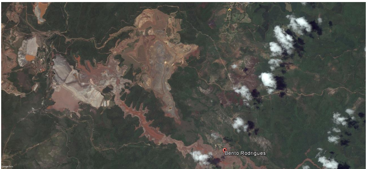
Figure 2: Fundão tailings dam from Google Earth immediately after collapse.
