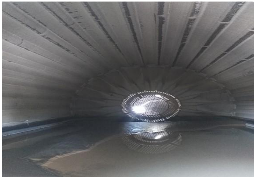
Figure 11: Ball mill discharge end after conversion.
