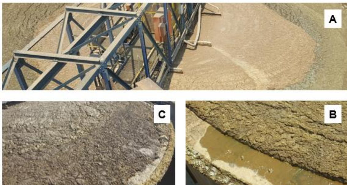
Figure 1: Froth covers the feedwell, launder and thickener surface and the fine particles it carries eventually block the launder.
