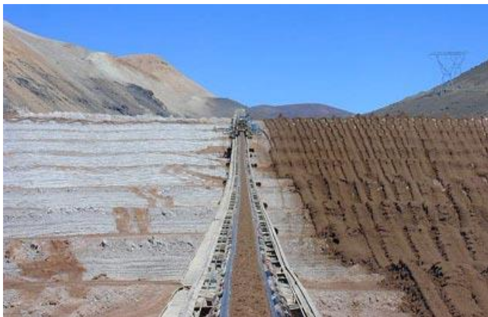
Figure 3: The "dry stack" tailings facility at La Coipa, Chile.
