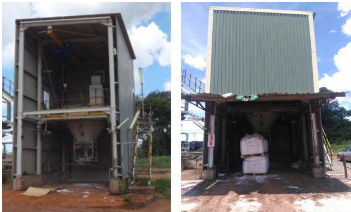
Figure 11: Flocculant building modifications.
