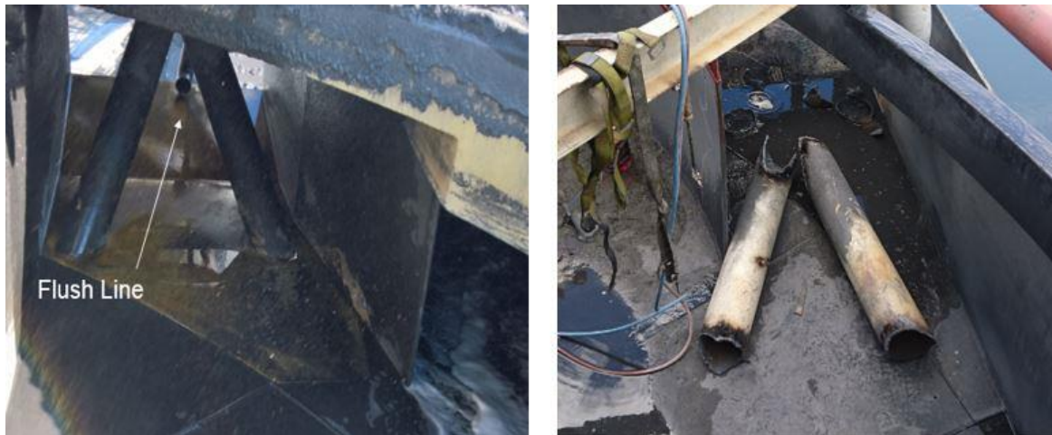
Figure 6: Channel mixing baffles.
