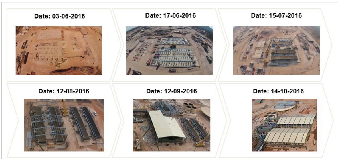
Figure 7: Boss 50 horizontal belt filter circuit and Kiwana thickener construction progression.
