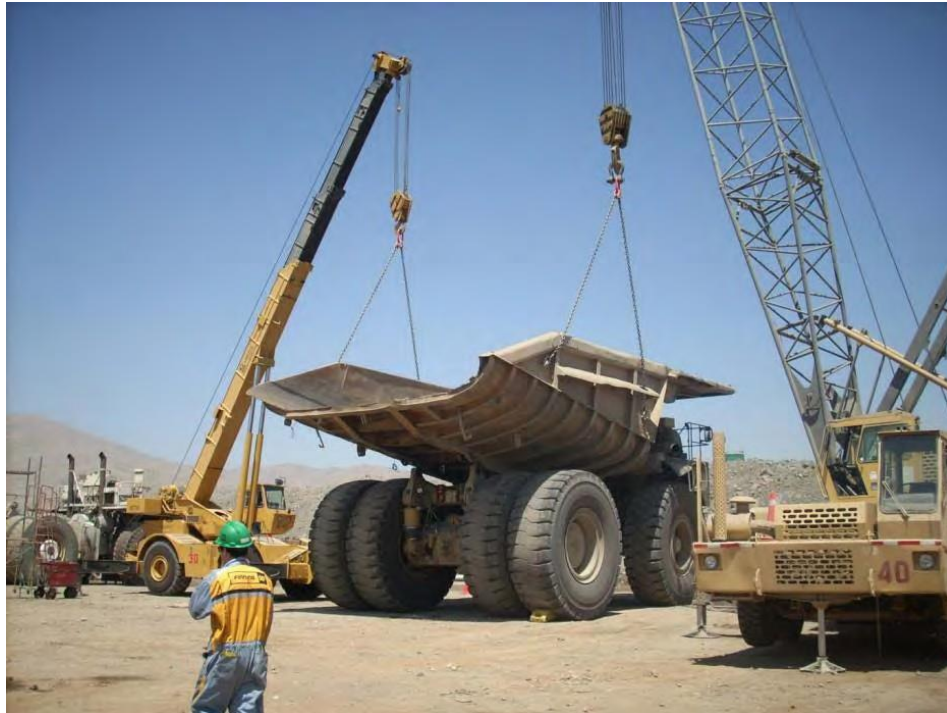
Figure 1. Typical method of dump body removal / installation executed with the use of two mobile cranes.
