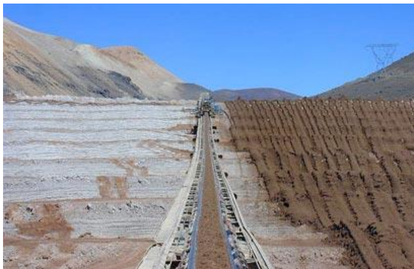
Figure 2. The "dry stack" tailings facility at La Coipa, Chile.
