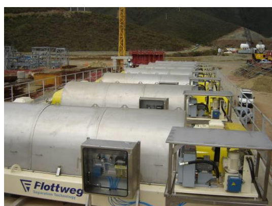
Figure 15. Centrifuge installation at Tiebaghi Nickel Mine in New Caledonia. (Photographs taken at Tiebaghi Nickel Mine, New Caledonia by Erwin Thalhammer, Flottweg SE.)
