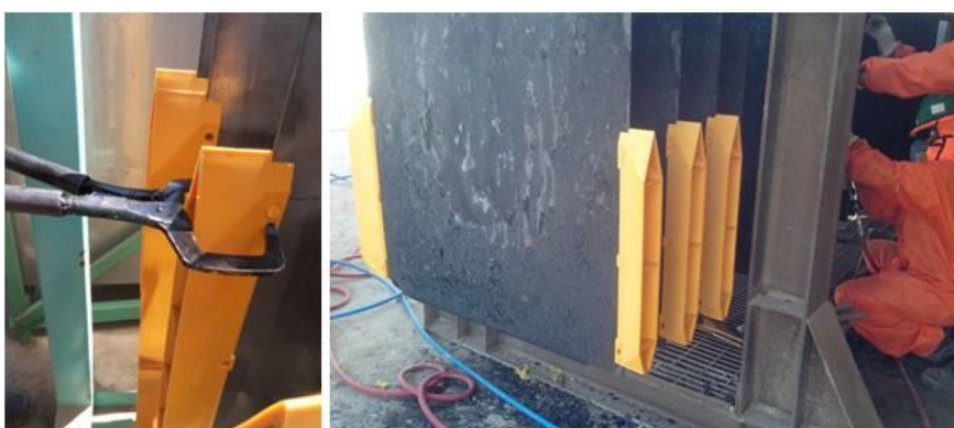
Figure 6. Installation of Idemin anode fittings at Lomas Bayas, Chile.
