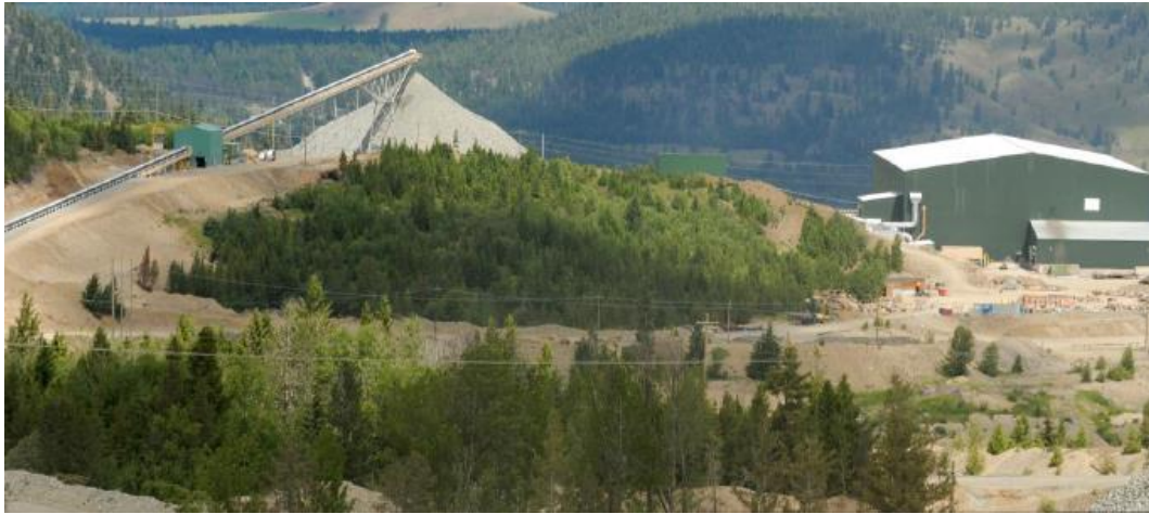
Figure 10. Original stockpile conveyor configuration with concentrator building on far right-hand side.
