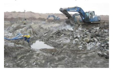
▶ Transvac Cleaning – cleaning the bedrock including cracks
