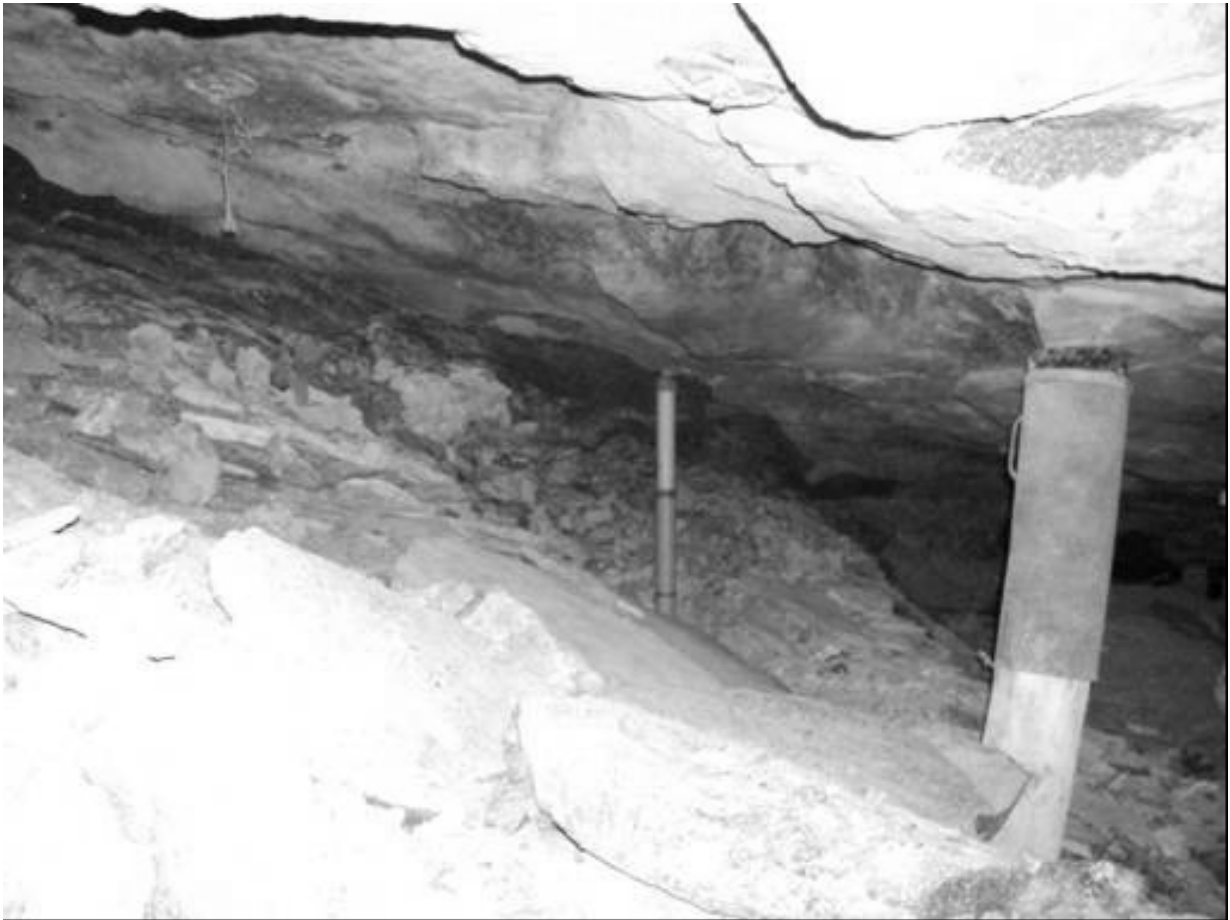
Figure 13 Down-dip side of the instrumented pillar. View away from face
