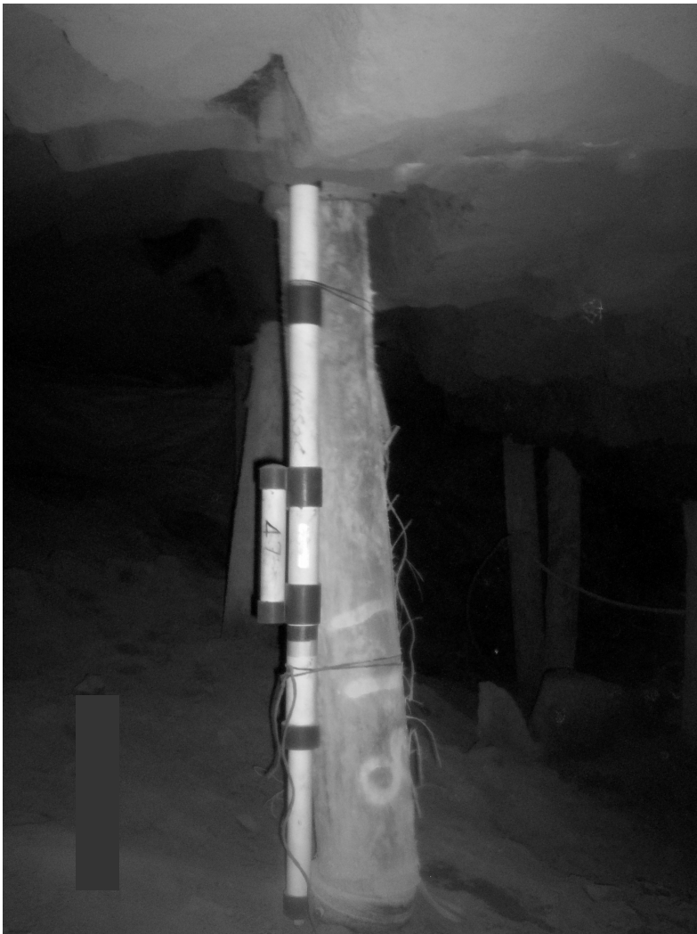
Figure 6. Closure and Load Loggers installed with a mine pole in a platinum mine
