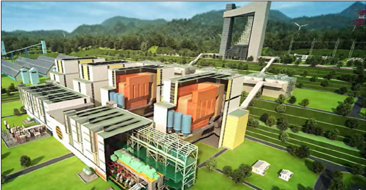
Figure 7. The Koso Samcheok project—4×550 MW el SC CFBs
