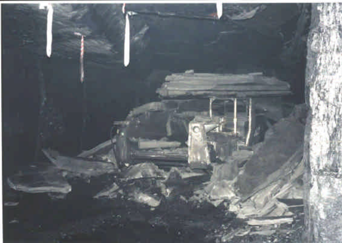
Massive roof fall along joint plane
