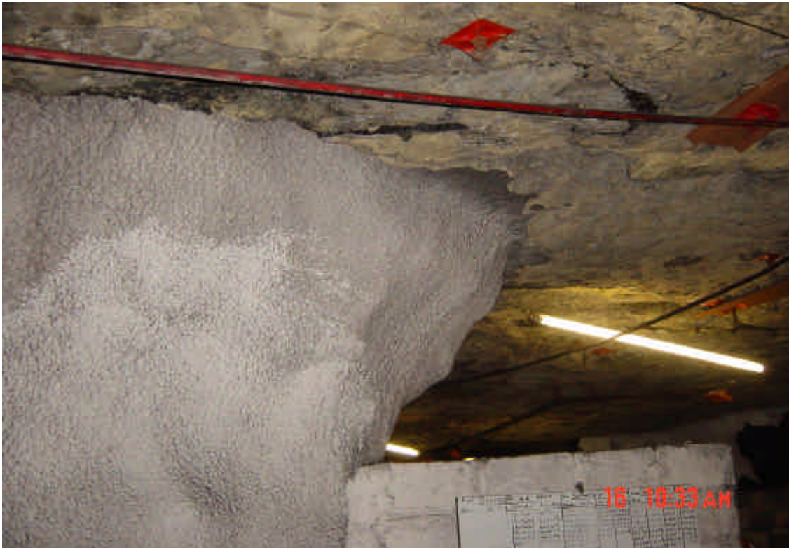
Mesh Covered with Shotcrete
