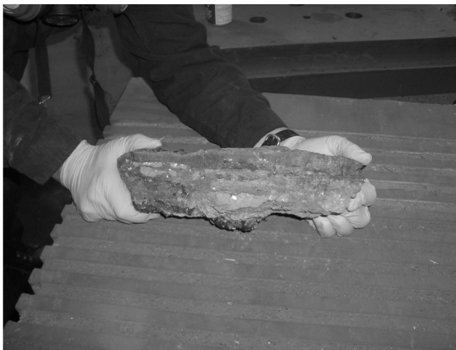
Figure 10. Spalled piece showing the layers of refractory, metal and accretion
