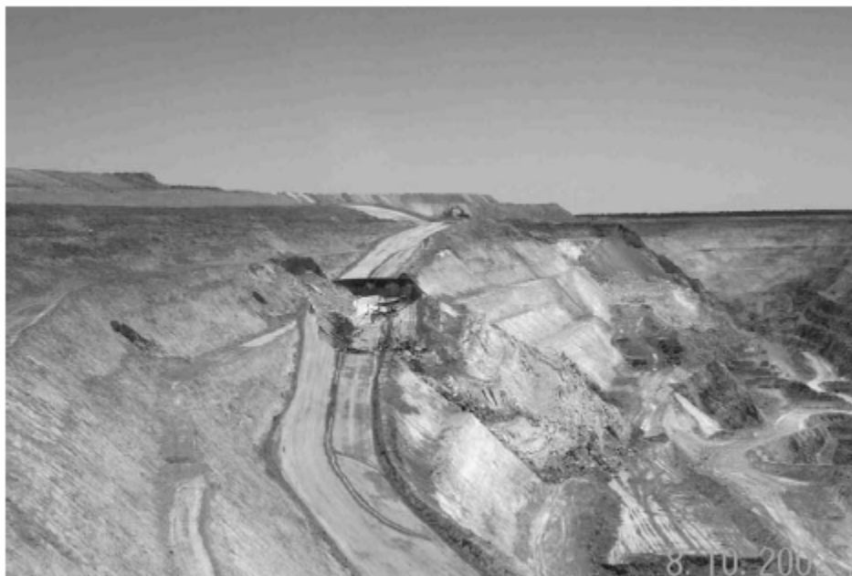
Figure 7 The Komatsu Ramp failure, Harmony Open Pit
