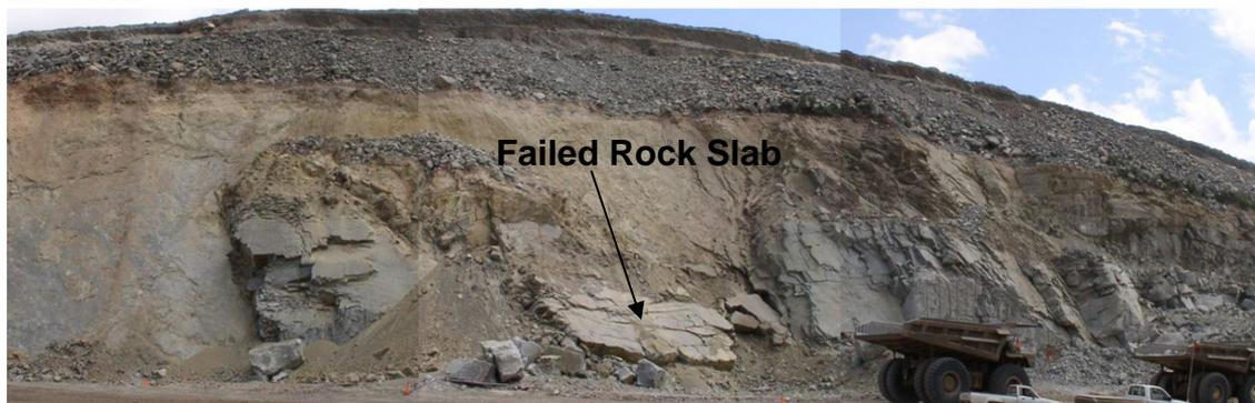
Figure 4: Small Rock Slab Failure
