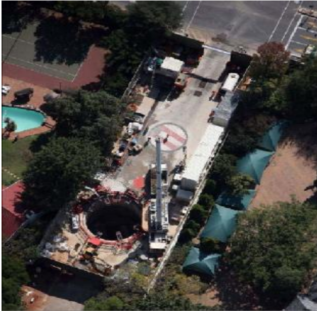
Figure 2 Emergency shaft E5, proximity to nearby residential property
