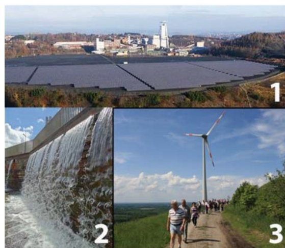
Figure 5. Creating renewable energy, an opportunity for post-mining. (1) Photovoltaic plant on a mud pond; (2) heat from mine water; (3) wind turbine on a dump.
