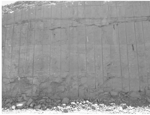
Figure 13: Level 950-935, Block AC 27-30 (Basalt, Splitex 32 mm Diameter)
