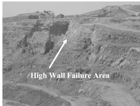
Figure 1: Orapa Mine high wall failure
