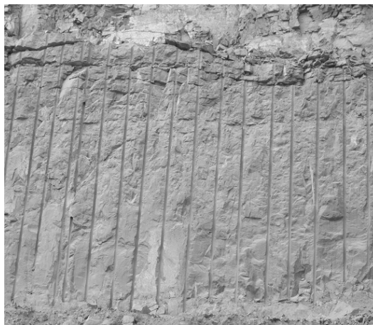
Figure 14: Level 935-920, Block ZAC 20-25 (Basalt, Splitex 32 mm diameter)
