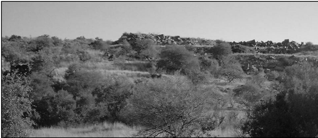
Figure 10 Terraced, topsoiled and rock shaded waste dump (Marikana Quarry)
