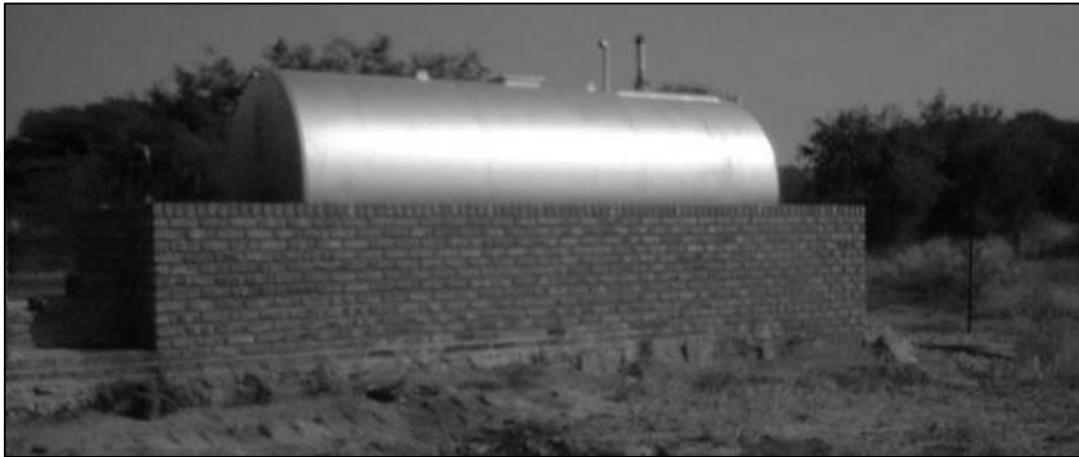
Figure 8 Bunded diesel storage facility (Nells Quarry)
