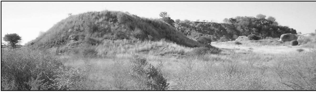
Figure 11 Waste dump covered with topsoil
