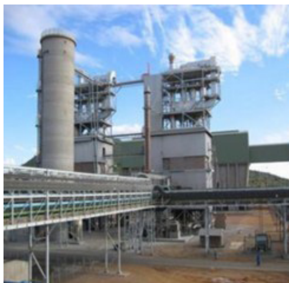
Figure 4—(left) Pelletising pans at the Waterval Smelter (after Mostert and Roberts, 1973); (right) Flash dryers and dry concentrate silo at Polokwane Smelter (Anglo American Platinum, 2016)
