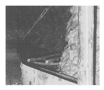
Figure 1—Shear zone observed in the sidewall of a footwall drive at a depth of about 2 km in the ERPM Gold Mine, South Africa. (Photograph by W.D. Ortlepp.)
