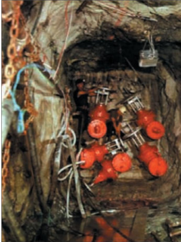
Figure 8—A long view of the main plug on 12 Level, illustrating the cramped space in which the men had to work when they ‘threw’ the plug. The television camera can be seen in the top right-hand corner to keep its eye on the first five valves
