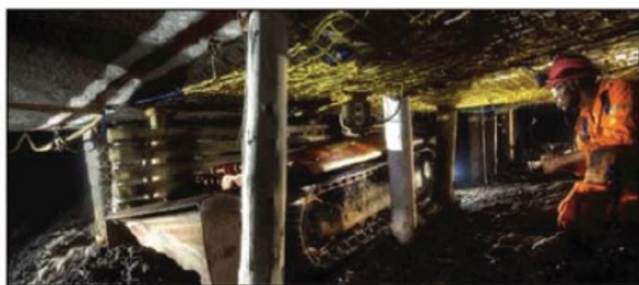
Figure 12—ULP dozer cleaning a panel (Fourie et al., 2017)
