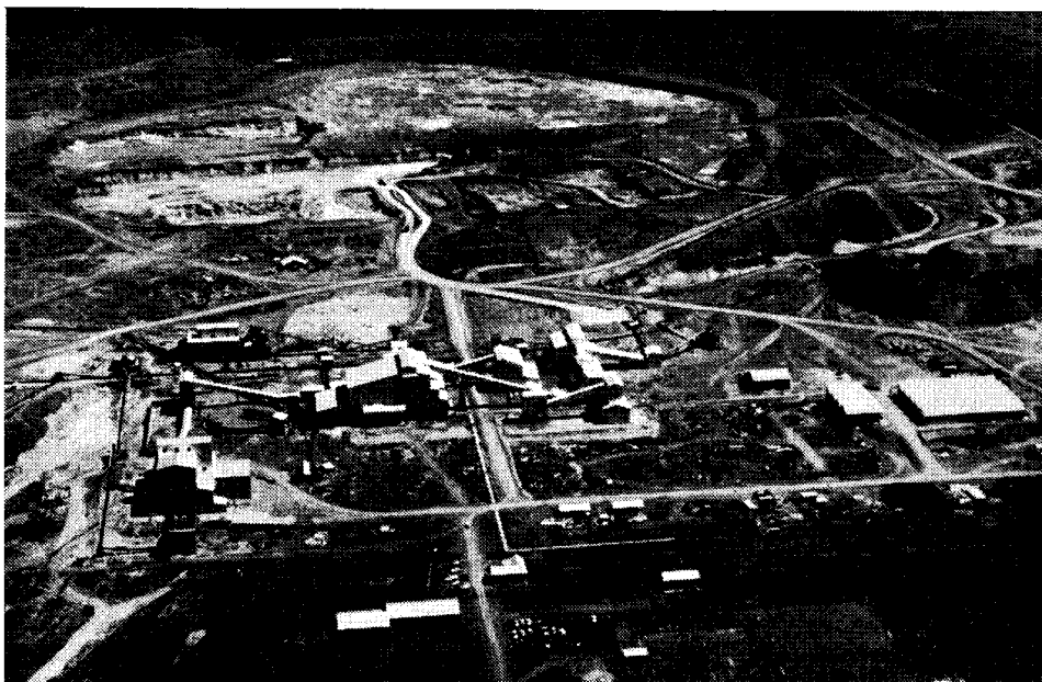
Fig. 11—A view of the mine taken early in 1966. The orebody has been fully exposed and the E-W face being established across the pipe can clearly be seen.
