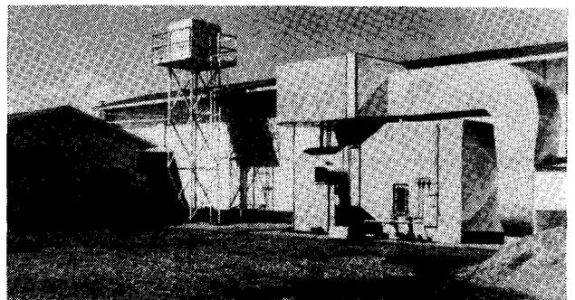
Fig. 1—Side view of a surface climatic room showing the machinery which automatically controls the temperature and humidity of the room
