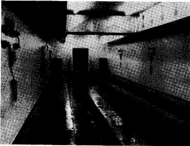
**Fig. 2—Interior view of the climatic room looking towards the stepping timetable flanked by two urinals in the corners. The long rows of stepping blocks can each accommodate 50 labourers. Note the specially designed air ducts in the ceiling**
