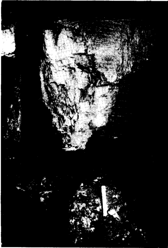
Fig. 11—Core of pillar after testing and barring, retaining sufficient residual strength to hang under its own weight.
