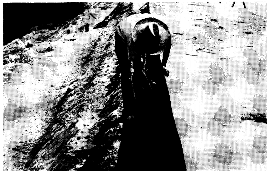
Plate IV—Disconnecting the steel plate
