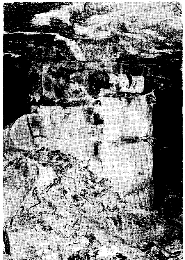
Fig. 2—The condition of a pack after the blast
