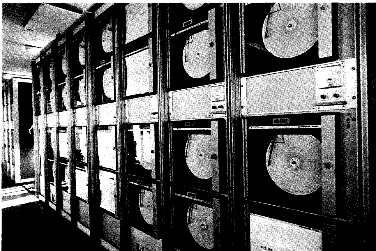
Fig. 6—A bank of separate 7-day chart records for the Spanair analysers and the Beacon detectors
