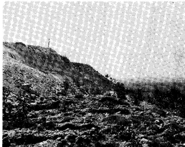
Fig. 13—Slickensided failure surface at Dump 5, indicating a 10 m downward slide of the material in the foreground
