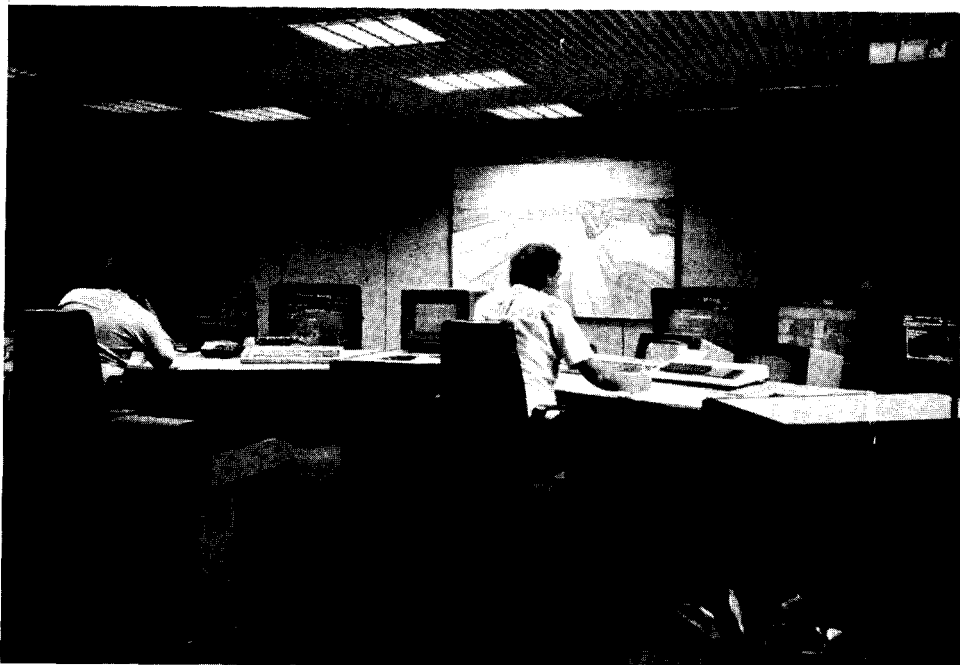
Fig. 1—The control room at Bergwerk Westerholt in West Germany (Photo: Bergwerk Westerholt)
