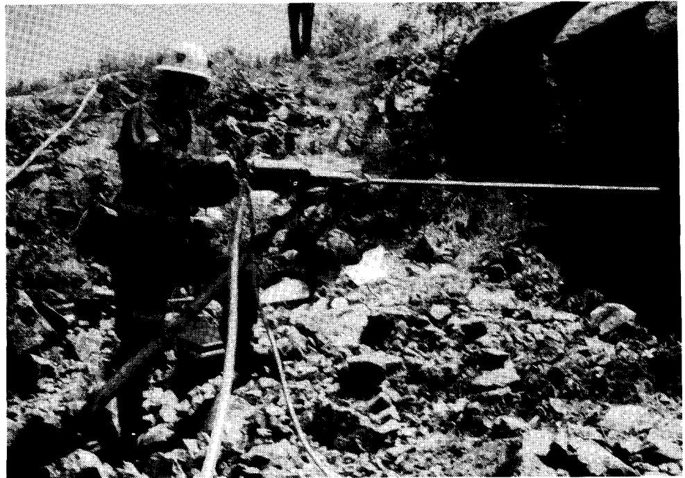
Fig. 2—The setup for the field test
