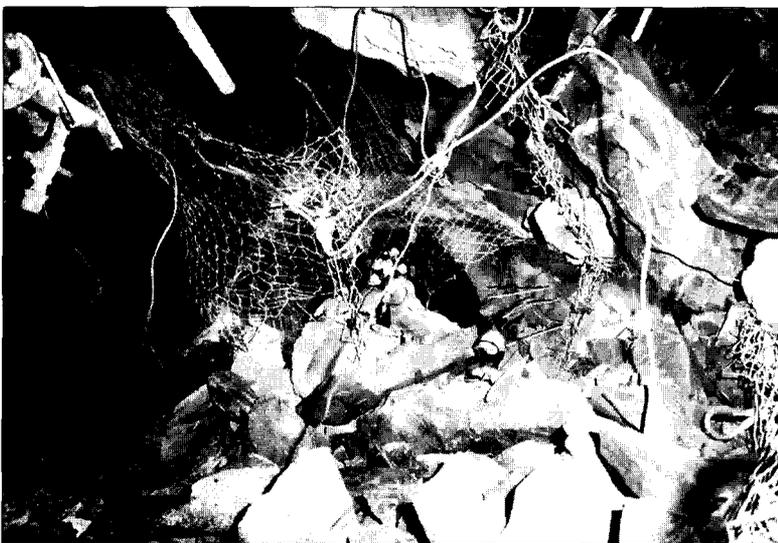
Figure 1—Damage to a tunnel supported by stiff grouted re-bar, mesh, and lacing after a moderate rockburst
