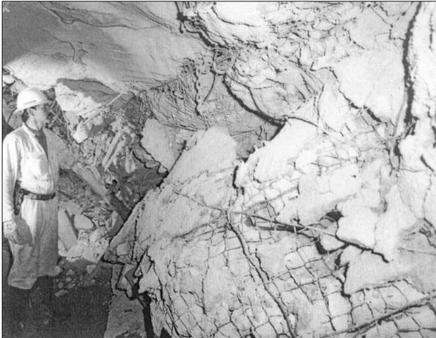
Figure 1—Support behaviour in a rockburst
