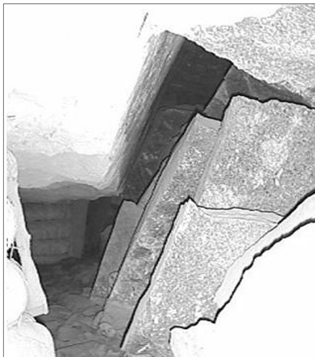
Figure 1—Photograph showing a major FOG from a smooth discontinuity with highly altered surfaces
