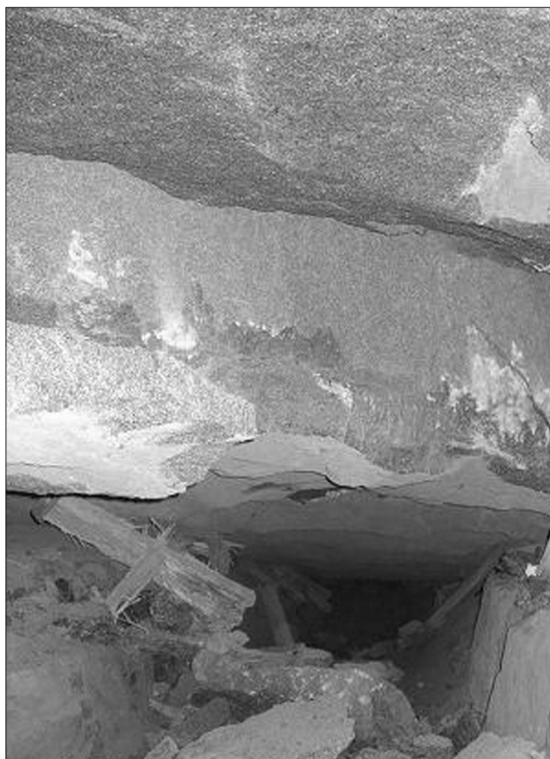
Figure 3—Photograph showing a collapse that occurred from a persistent, unfavourably orientated joint (Watson, 2003)
