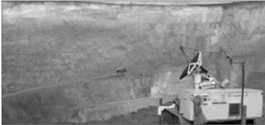
Figure 5—Groundprobe's slope stability radar, monitoring the south east wall at Harmony
