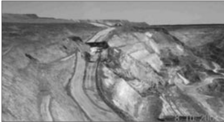
Figure 7—The Komatsu ramp failure, Harmony open pit
