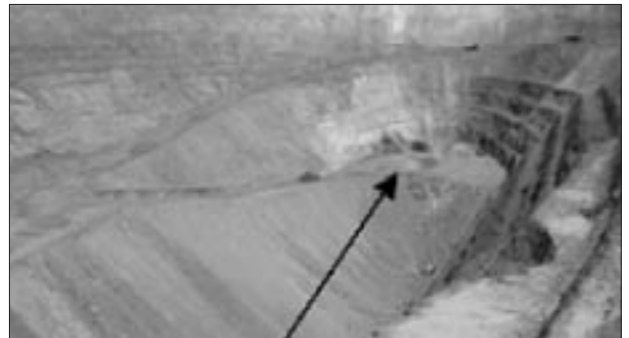
Figure 13—Excavation has advanced 30 m in depth
