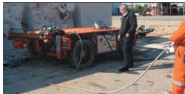
Figure 10—Face drill carrying out test drilling
