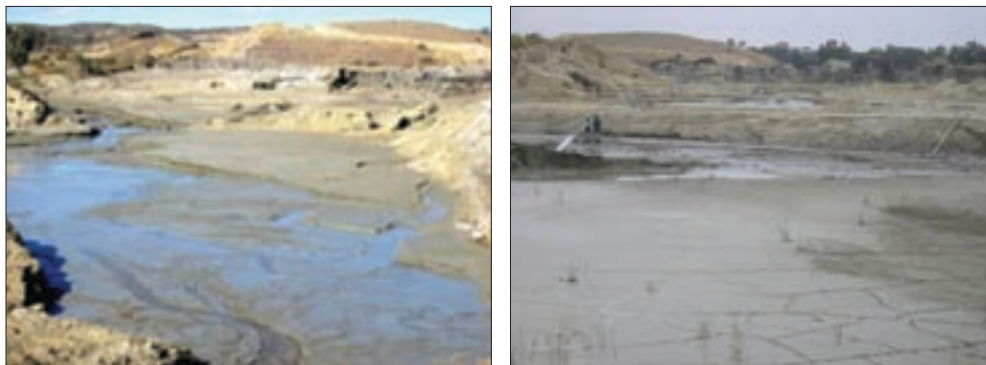
Figure 7—In-flow to tailings dam pump station with tailings dams in background and view of the Klipfontein pump station and inlet area
