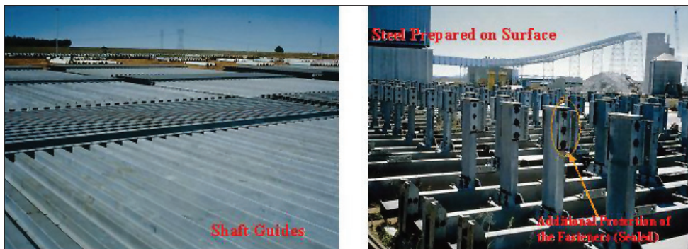
Figure 5—Hot dip galvanized steelwork waiting to be transported underground (1992)
