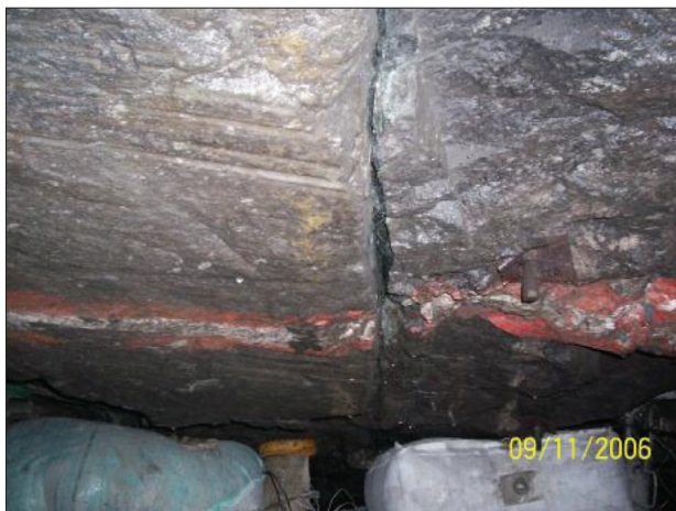
Figure 3—Opening of a discontinuity in one of the ASDs at the Declines Section
