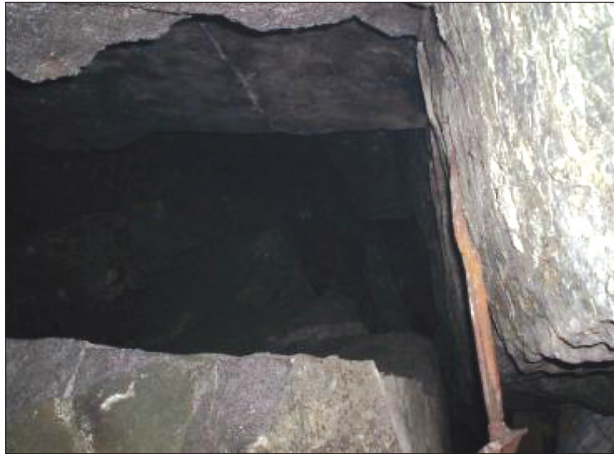
Figure 1—Planar nature of the steep dipping joints as exposed by a large fall in Panel 15S, 4S decline
