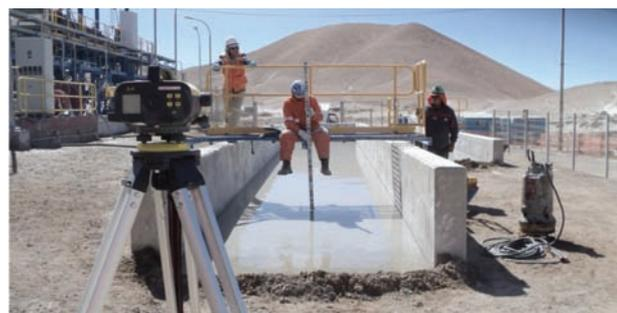
Figure 3—Measurements within the larger flume
