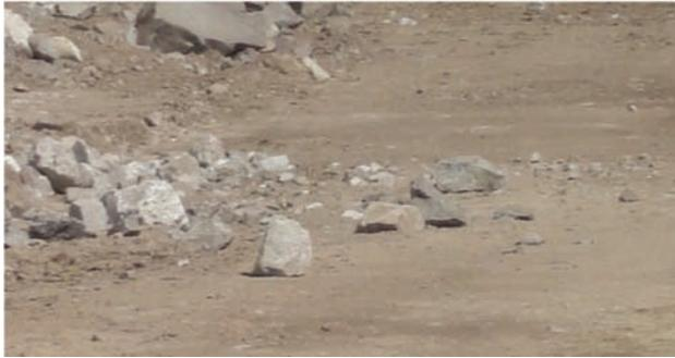
Figure 10—Example of spillage on the in-pit haul road
