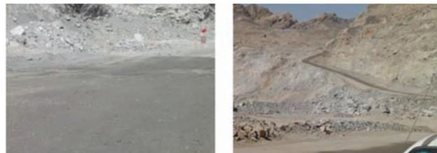
Figure 9—Undulation of in-pit haul roads at Rössing
