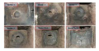
Figure 14-Cold face of tapping modules
