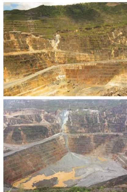
Figure 11—Erosion effects of extreme rainfall, before (above) and after (below). Photographs courtesy of John Read
