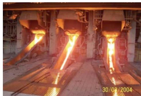
Figure 1—All three slag tap-holes open with near-continuous slag tapping on a PGM matte furnace. Notice hood extraction
