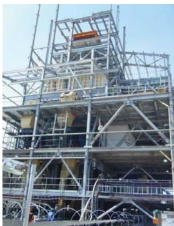
Figure 8—Karowe's XRT section during construction in Q2 2015
